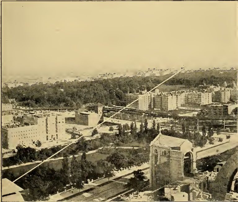
NEW HARLEM LINE FROM THE NORTH.
